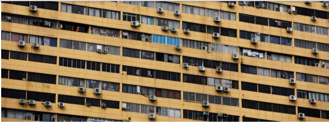
Air-conditioning units dot the facade of an apartment block in Singapore. Photo by Edgar Su/Reuters
